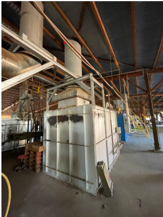
Image 2. MP3 - Afterburner of Propellant Furnace
